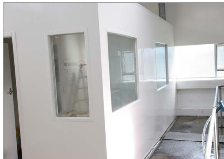
Formwall installation showing smooth, thermoformed external corner and formed window insets.
