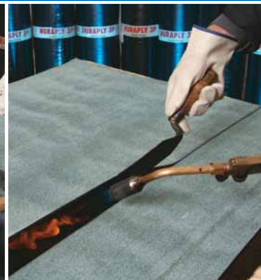
C - Welding lap joints
