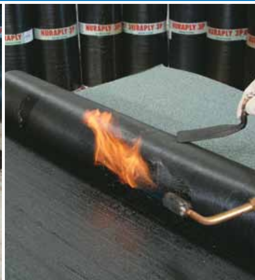
B - Melting off protective sheet
